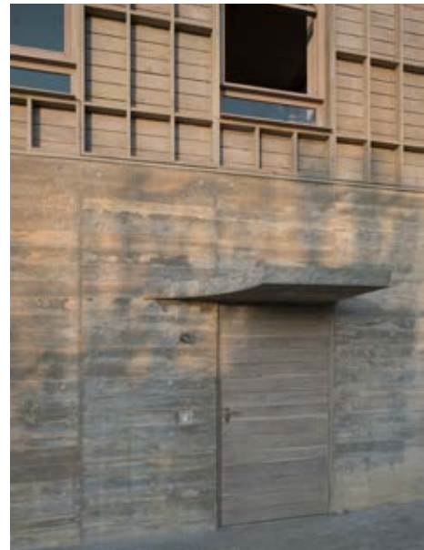
Figure 3c: Pine Concrete House.
